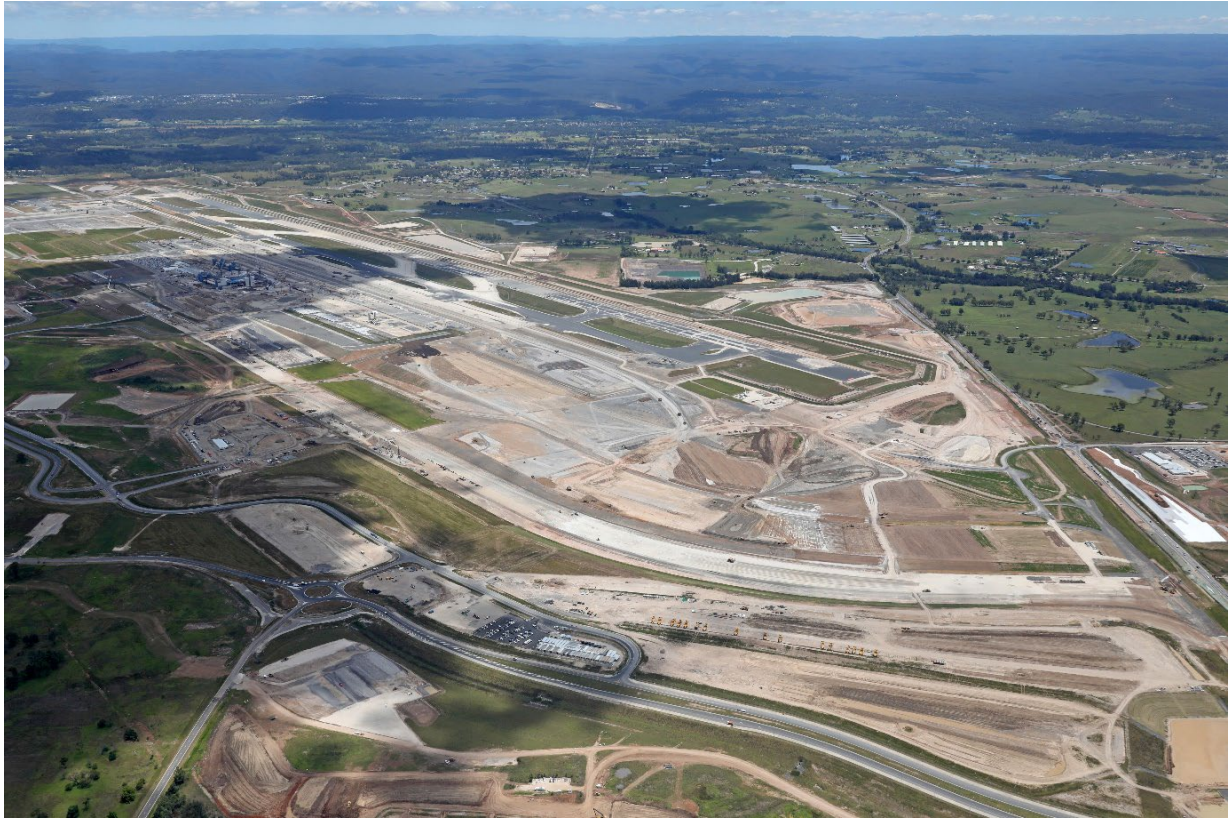
Construction underway on Western Sydney International (Nancy-Bird Walton) Airport.
