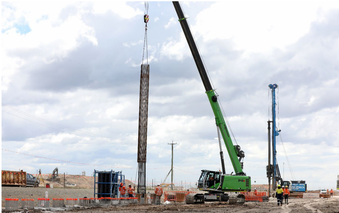
Construction at Airport Terminal site.
