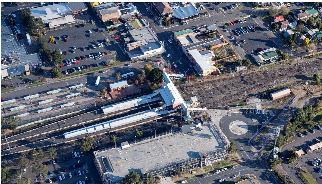
Aerial view of St Marys station.
