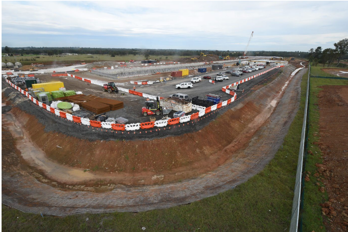
Construction at Aerotropolis site.
