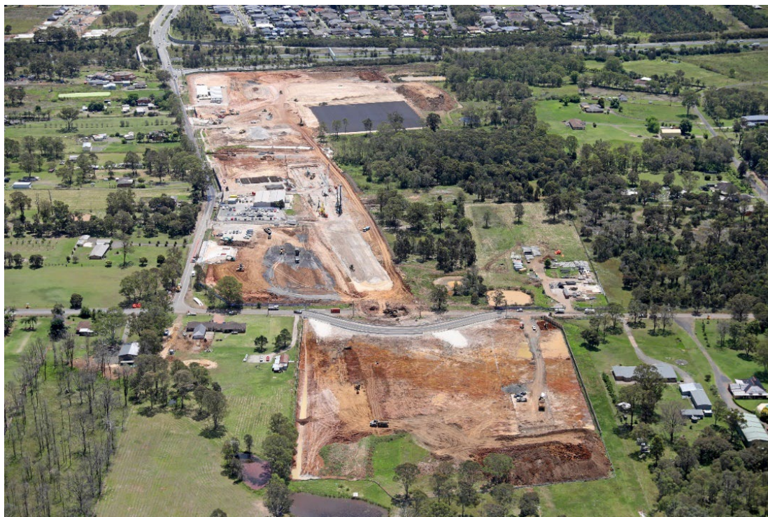
Construction at Orchard Hills site.
