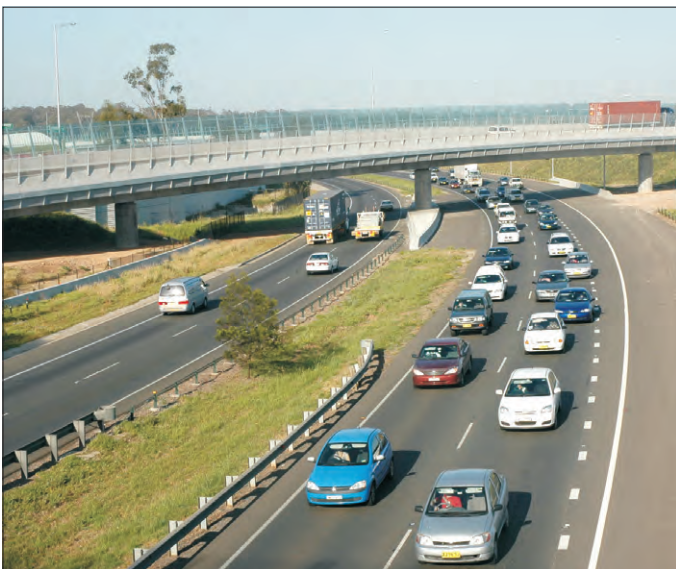
The same view in 2006, following the completion of the interchange with the Westlink M7 motorway, previously known as the Western Sydney Orbital, in late 2005. The flyover shown here is a ramp from the southwestbound M5 to the northbound M7.
