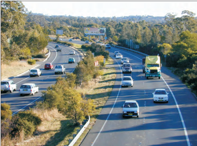
Looking southwest in 2002 from the Beech Road bridge over the M5 in Casula, on the “M5 Western Link” section of the motorway constructed in 1993–94.
