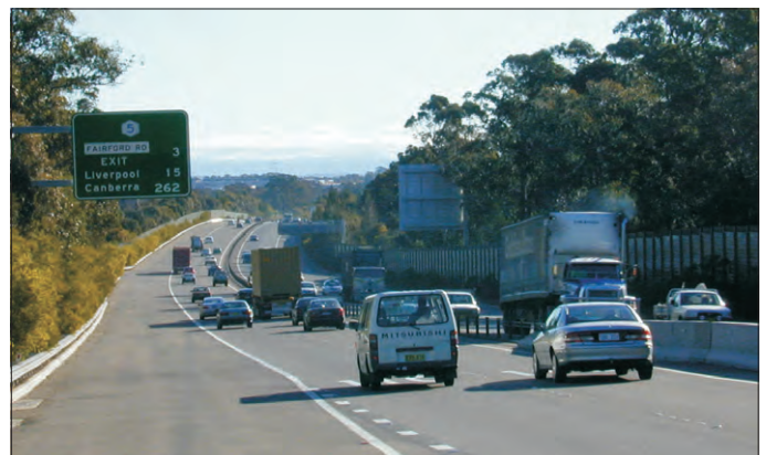
Looking west from the bridge over Penshurst Road, Narwee, on the King Georges Road–Fairford Road section of the motorway duplicated in 1997–99.
