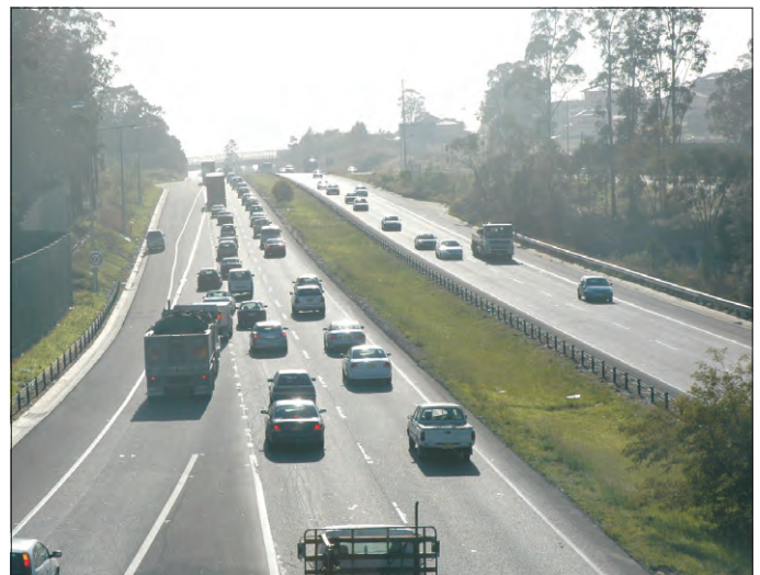
The same view in 2006, following the completion in late 2005 of new off-ramps for southwestbound M5 traffic to Beech Road and the northbound Westlink M7 motorway, just visible on the right of this photograph, and a new on-ramp from the southbound M7 to the northeastbound M5, at left.
