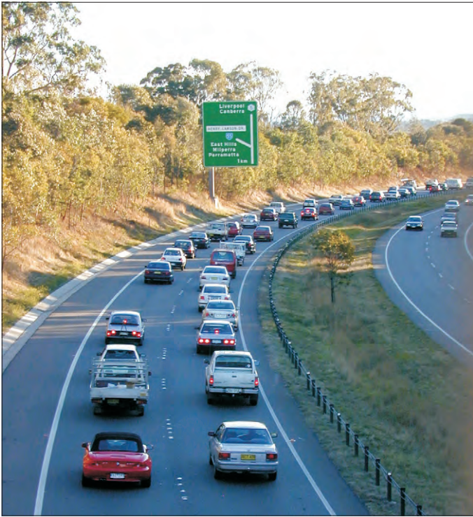
Looking southwest from the Beaconsfield Street bridge over the M5 in Revesby, on the original Stage 1 section of the motorway constructed in 1991–92.
