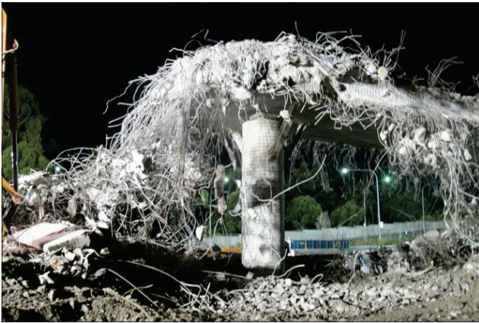
Demolition of the busway from the M2 motorway to Epping station.
