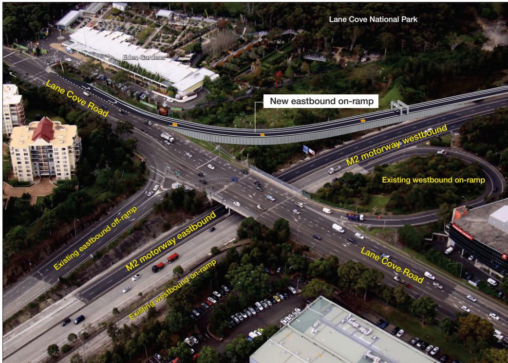
Figure 1.6. The new eastbound on-ramp from Lane Cove Road to the M2 motorway in Macquarie Park.
