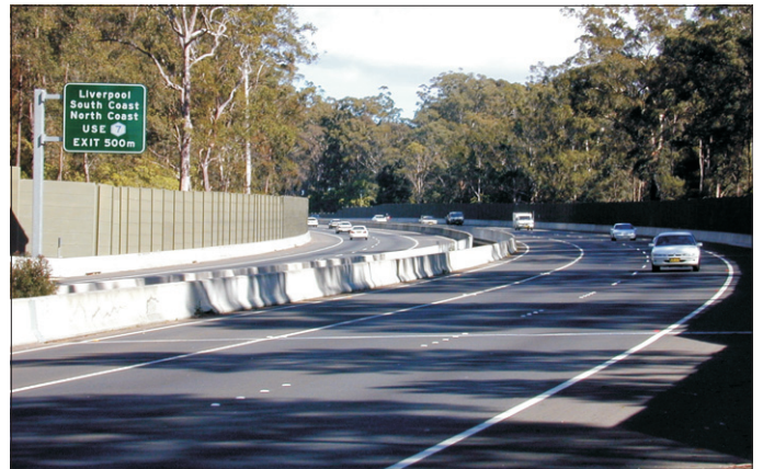
Devlins Creek bridge, Beecroft, in 1999.
