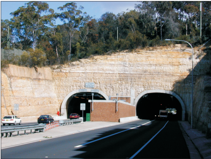
Eastern portals of the M2 tunnels under Norfolk Road, Epping, in 1999.
