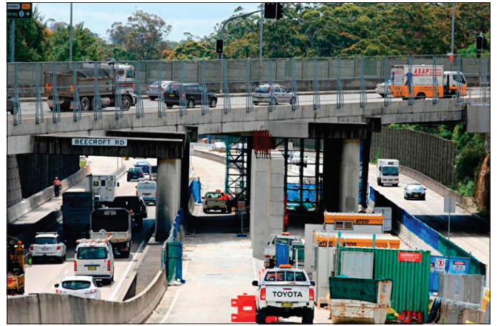
Beecroft Road overpass works in December 2011.
