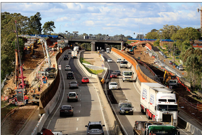
Works for the new west-facing ramps at Windsor Road in June 2011.
