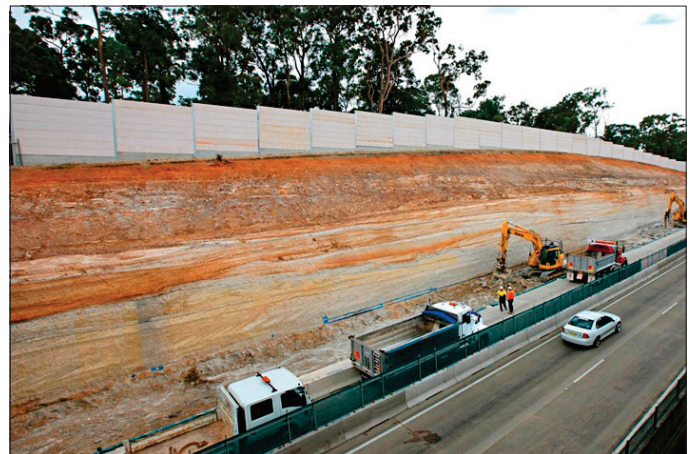
Excavations east of the Barclay Road overpass in December 2011.
