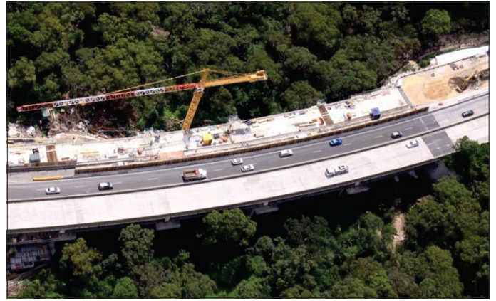
Widening of the Terrys Creek bridge in February 2012.
