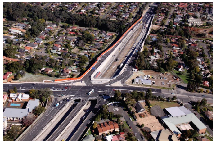
The Windsor Road interchange, looking west, in July 2012.
