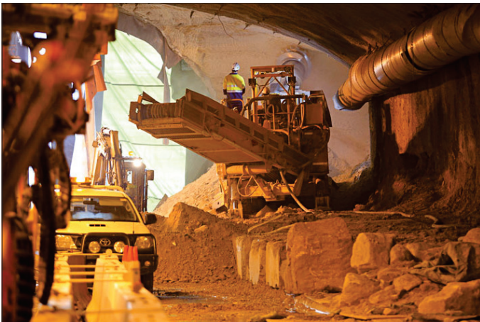
Widening of the M2 tunnels under Norfolk Road, Epping, early in 2012.
