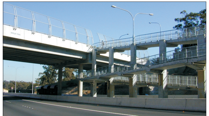
Barclay Road bridge and bus stop, North Rocks, in 1999.
